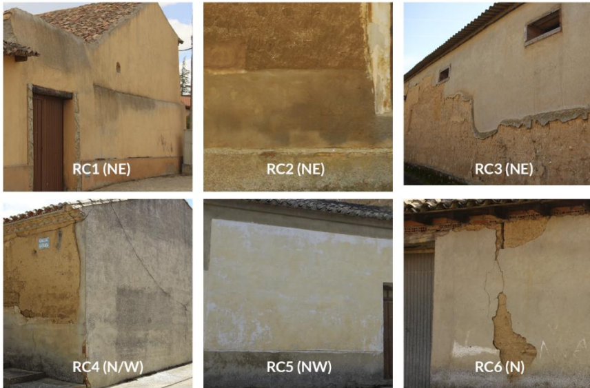
Figure 3: Photographs of north, west, northwest and northeast orientation
