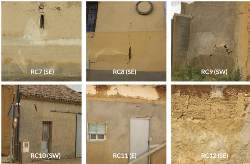
Figure 4: Photographs of south, east, southwest and southeast orientations
