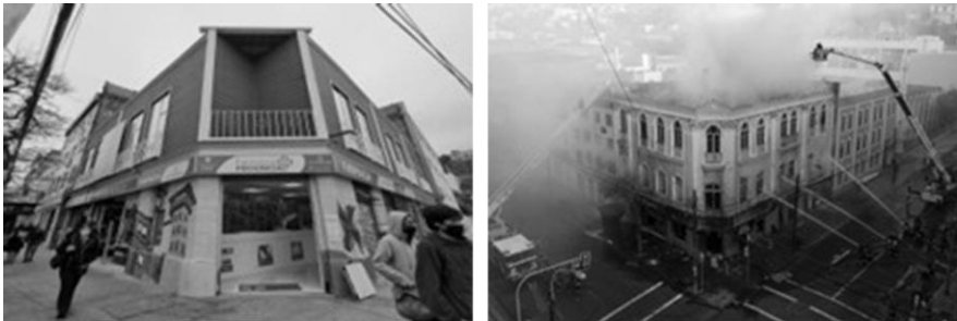
Figure 2: Pre- and post-fire comparison of the property. Source. Left www.bbc.com . BBC, 2019. Right. Author, 2023
